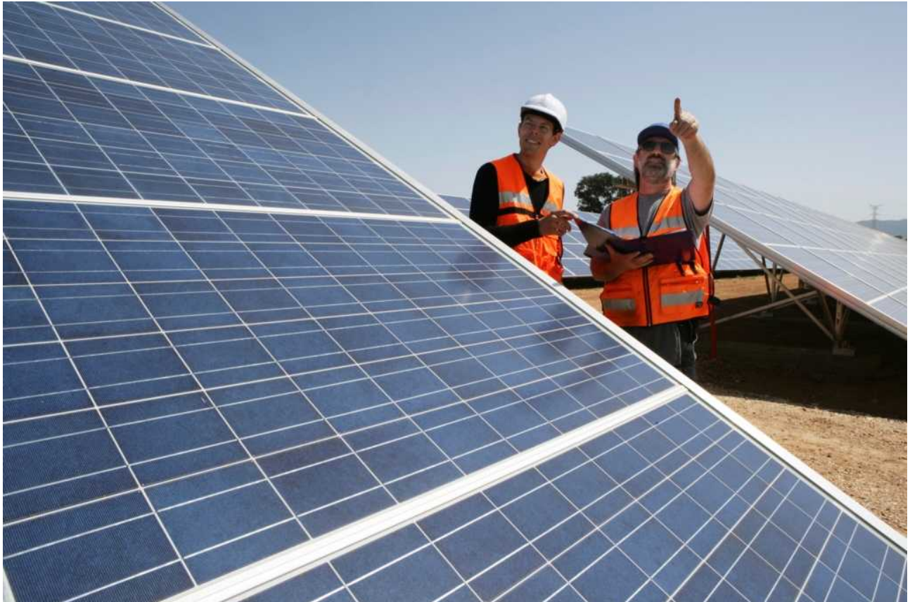
A solar power plant in Beneixama, Valencian Community, Spain. [picture alliance / imageBROKER | Jochen Tack]
