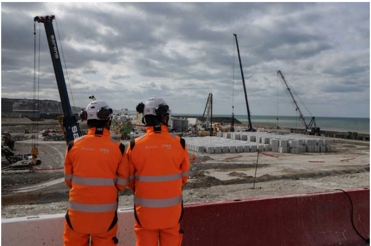
Workers look out at the EPR2 construction site of the new reactors currently being built at the Penly nuclear power plant in Petit-Caux, France, March 12, 2026. picture alliance | LUDOVIC MARIN
